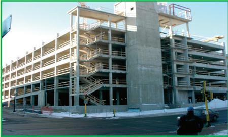
An 1,800 vehicle, six-level parking garage needed all of its 22,000 cubic yards of concrete to meet or exceed 3,000 psi strength within 18 to 24 hours.
